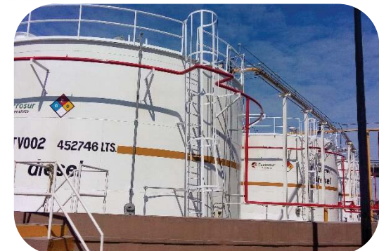
PROTECTION AGAINST UV RAY DAMAGE
